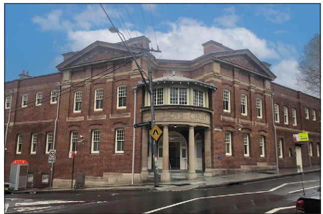
Surry Hills Children's Court 66-78 Albion Street, Surry Hills
