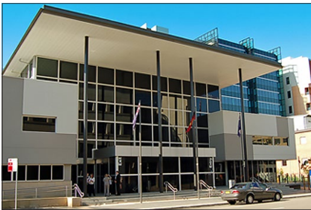
Parramatta Children's Court 2 George Street, Parramatta
