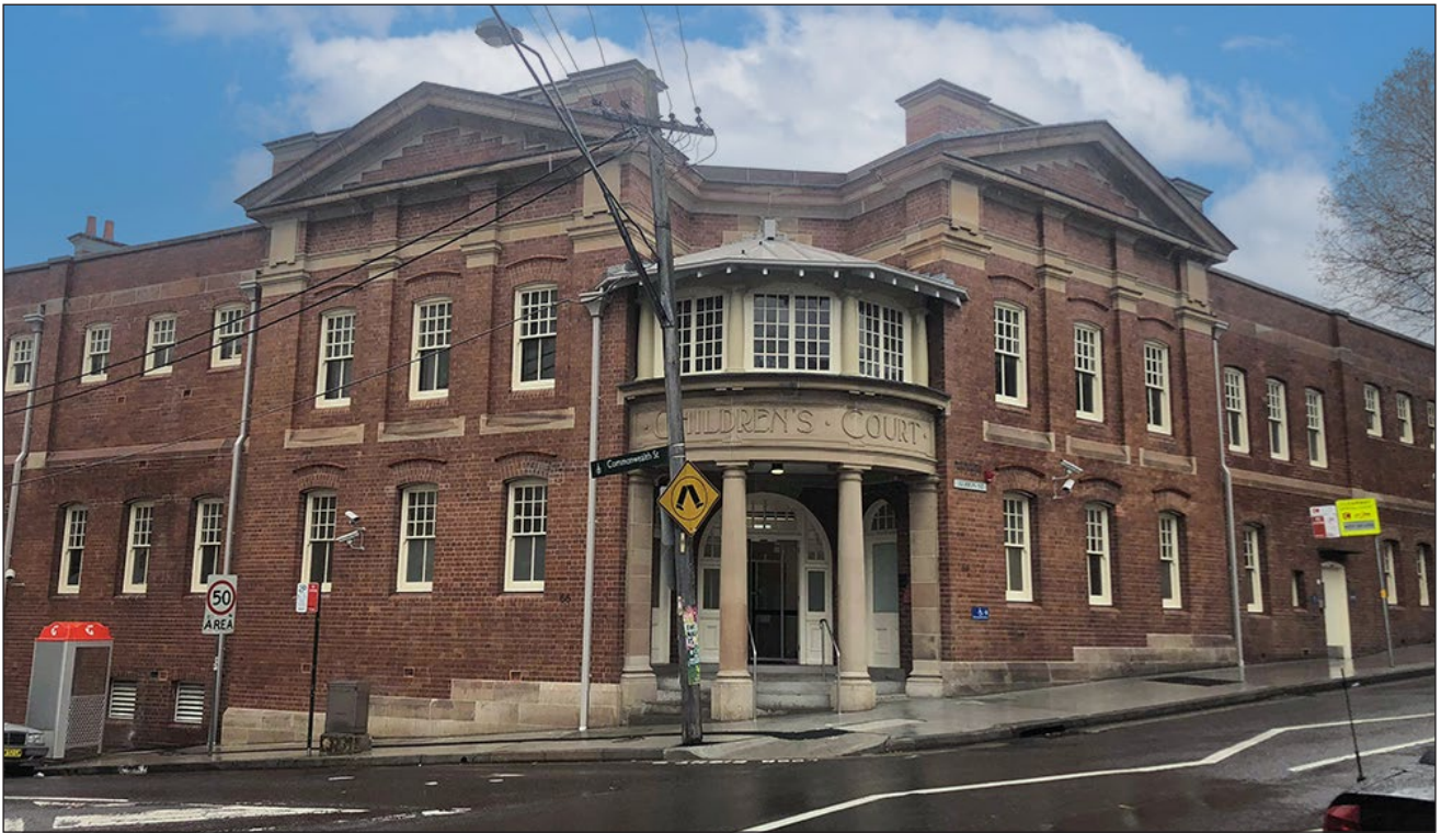
Surry Hills Children's Court, 66-78 Albion Street, Surry Hills
